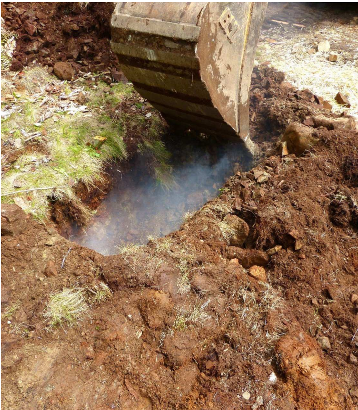
We dug holes for the poles,
