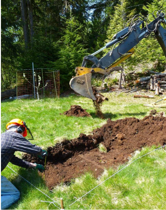
Phil measures the trench making sure we get 2 1/2 feet.
