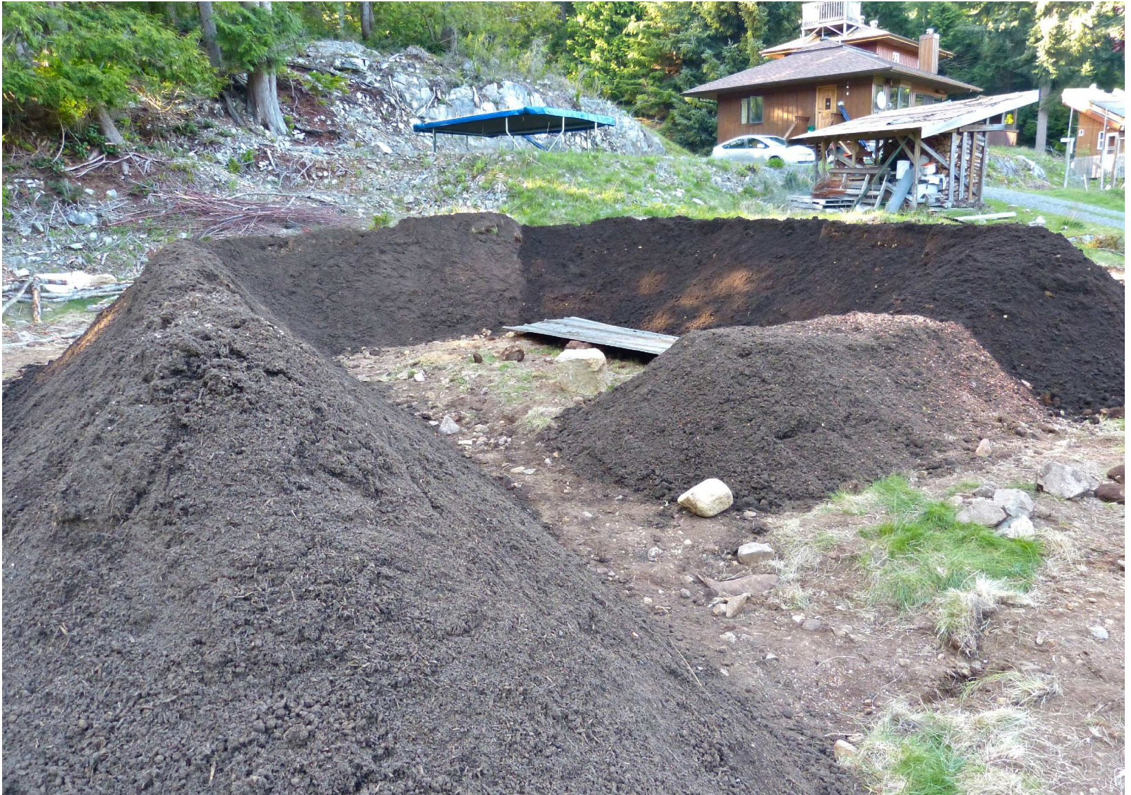
Soil all on and ready for more planting.
